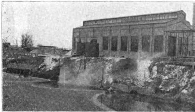
View of Walnut Creek Power Station from River Side Showing Intake and Discharge Water Funnels, Feed Water Purifying Plant and Portion of Outdoor 39,400-Volt Bus Structure.
